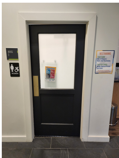
First Floor Bathroom Door
